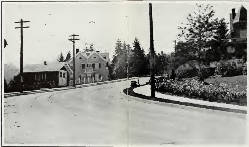
Hassam Pavement, Vista Avenue, Portland, Oregon. The portion of the street occupied by the streetcar tracks is also paved with "Hassam"
